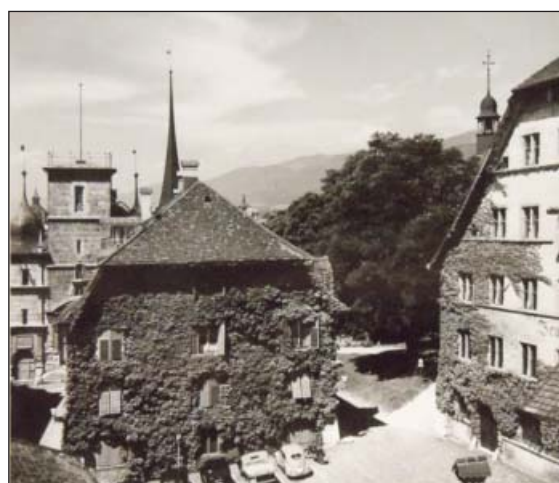
Fig. 4: In 1905, Arthur Gloor moved his practice and his family into this huge house on the same street as the city hall («Rathausgasse 17»), which was built before 1538. Behind is the Renaissance city hall, and on the right the armory («Zeughhaus»)
